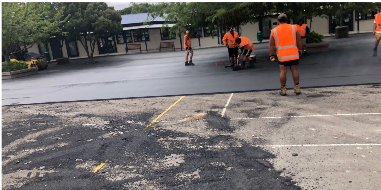
Contractors laying the new surface for the Hadlow Quad
